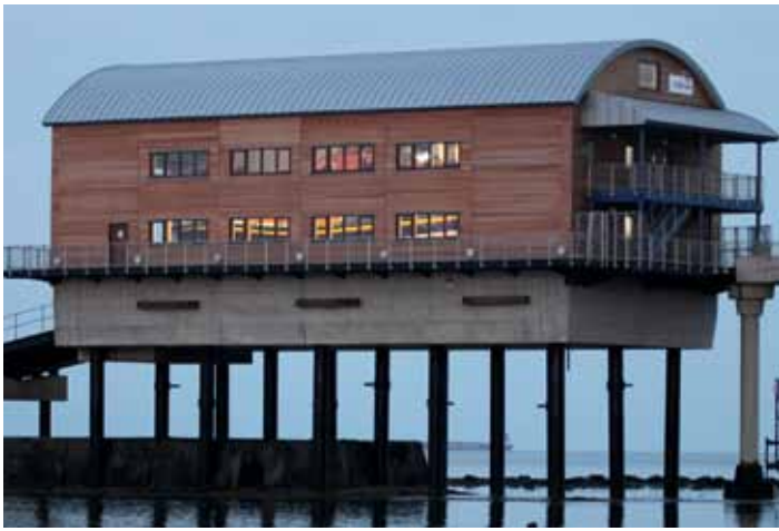
The new Bembridge Life Boat Station
